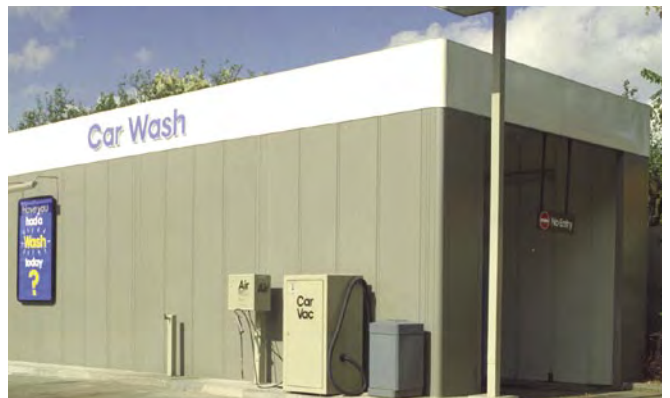
A wash housing is constructed using COMPOSOLITE® 3-way connectors, toggles and panels. No internal structure is required. Dimensions are 36' x 16' x 14'-3/4" (11m x 4.88m x 4.29m) high. Low maintenance, ease of construction and an attractive appearance greatly benefited the customer.
