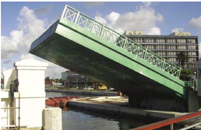
An all-composite bascule bridge in Bridgetown, Barbados, was built using Strongwell's COMPOSOLITE® building panel system, EXTREN® structural shapes and a custom heavy-duty building panel. The drawbridge is mainly used by pedestrians in this tourist destination, but it is also designed to support vehicular traffic.
