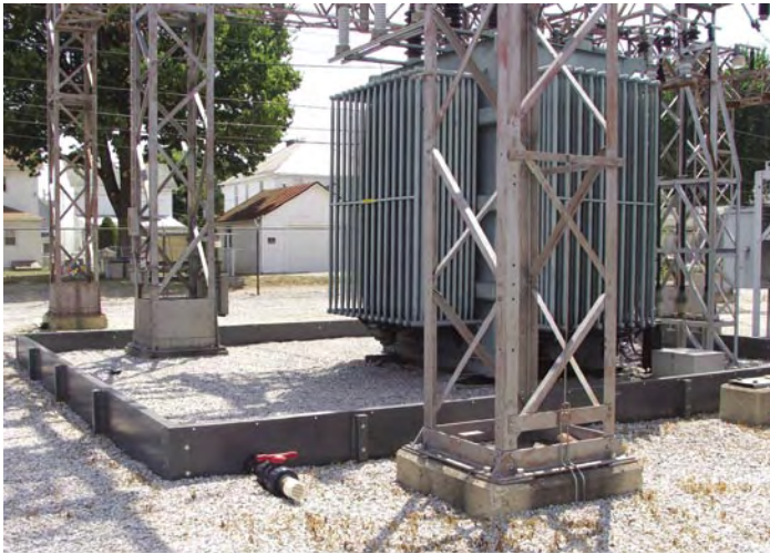
An oil containment system using COMPOSOLITE® surrounds a transformer at this electric utility substation. Compared to concrete or earthen containment systems, the COMPOSOLITE® system saves time and money during installation.
