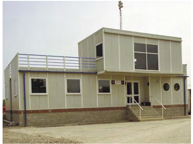
A visitor center in Bristol, UK, is constructed of COMPOSOLITE® panels, 3-way connectors and toggles with no supporting frame. Cells of panels and 3-way connectors were filled with foam for thermal insulation.
