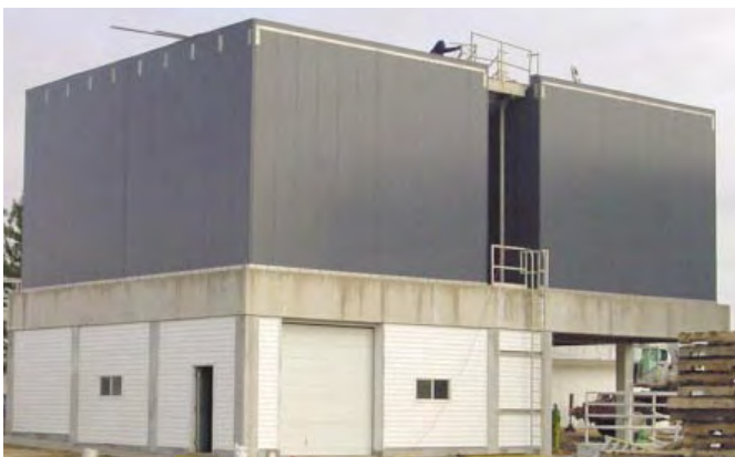
The Lexington Waste Water Treatment Plant used COMPOSOLITE® panels to refurbish its above-ground trickling filters. COMPOSOLITE® was chosen because of its corrosion resistance, ease of installation and long-term reduced maintenance cost.
