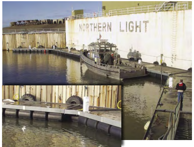
A removable dock system featuring lightweight, corrosion resistant COMPOSOLITE® panels and EXTREN® structural shapes is located on the Baufort Sea. The sea freezes in winter, making easy removal of dock sections a necessity for the customer. Each section is 12' wide by 30' (3.66m x 9.14m) long.
